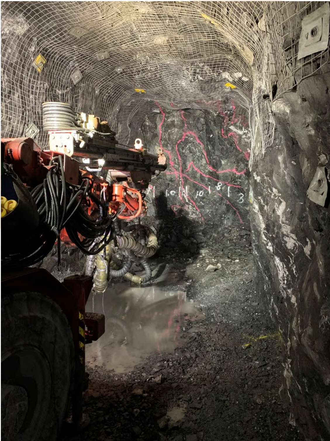
Ore drive underground at Golden Eagle
